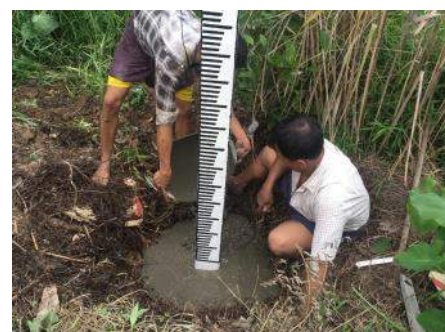
Installing water level measurement gauge
